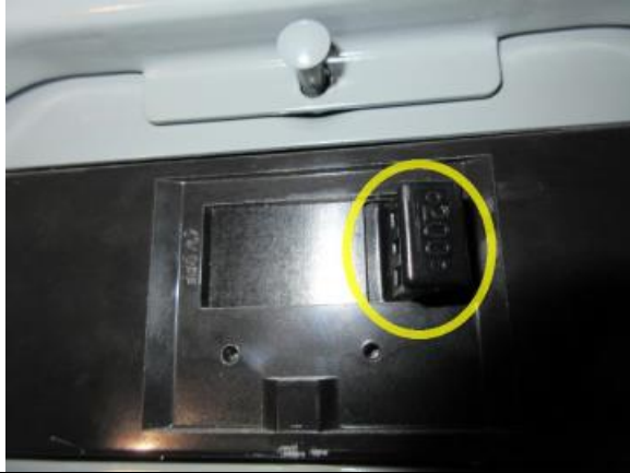
8.5 Service Disconnect Switch: Located at the top of main panel.
